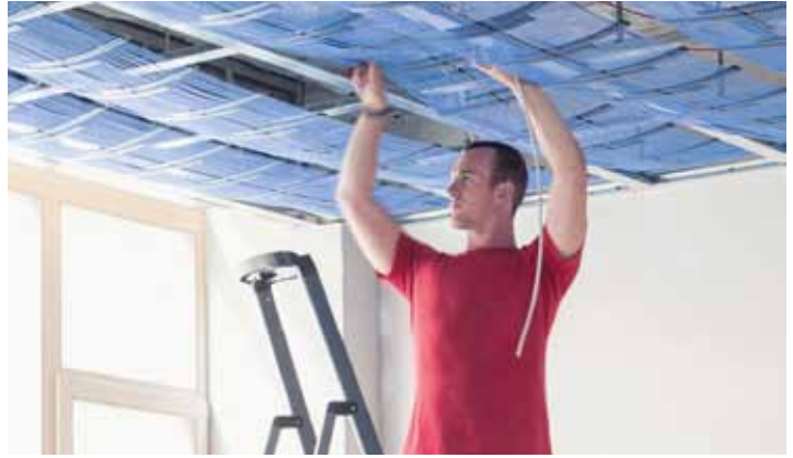
Capillary tube system by GeoClimaDesign as overhead heating and cooling system
